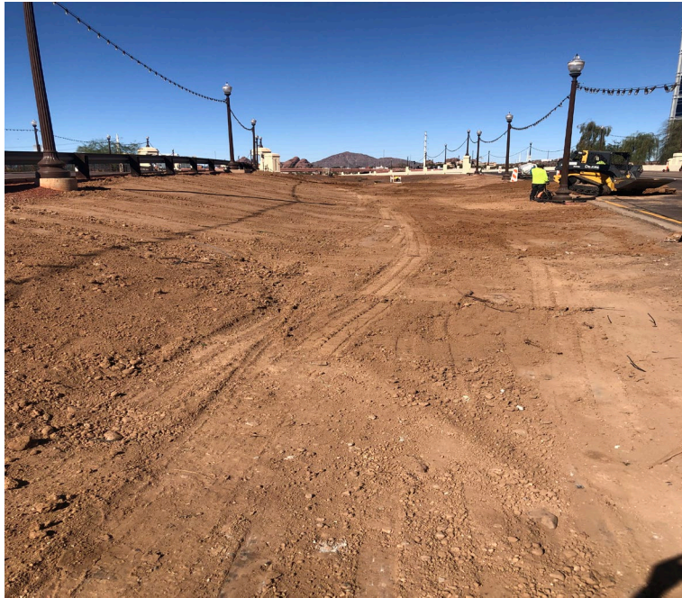
Mill Ave Bridge before and after
