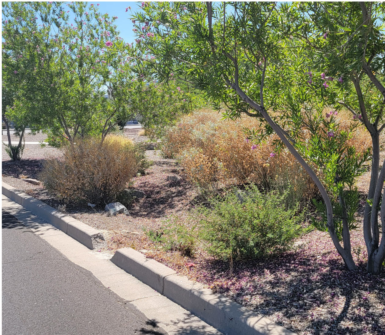
Figure 7-1: Potential offsite stormwater credit for bioswale in the ROW in Tempe, AZ
