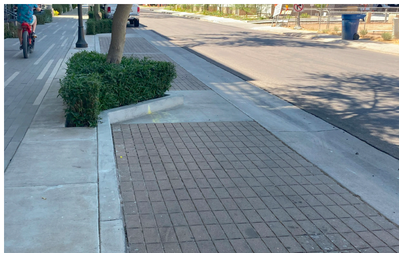
Figure 7-2: Potential offsite stormwater credit for permeable pavers in the ROW in Tempe, AZ
