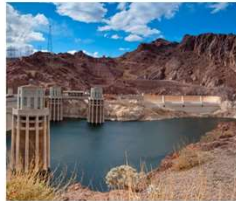
Severe Drought & Water Use
