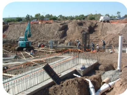
Early work on the TCA, such as pouring footings and installing utilities, has been underground.
