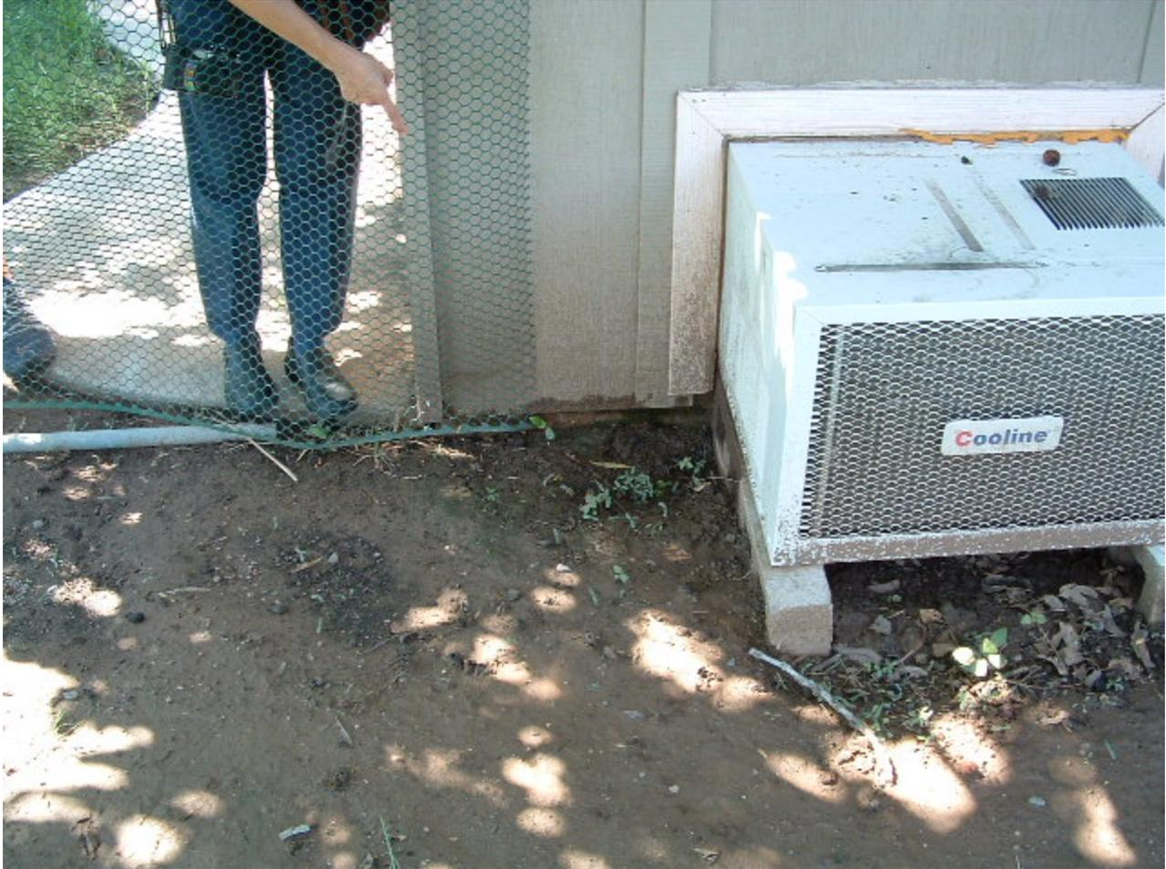
The corner of this house has no berm to prevent water from contacting the structure. As the water reaches the same level as the foundation, it seeps in behind the exterior wall, leading to extensive damage over time.
